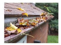
Some of the units have tons of leaves in the gutters. This not only looks bad but can cause damage to roof and lanai.
