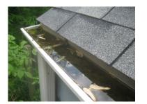
Some units have branches and weeds growing out of the gutters. This causes damage to the roof itself.
